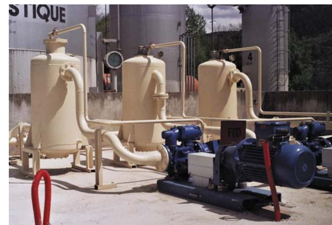
Caustic soda Transfer
